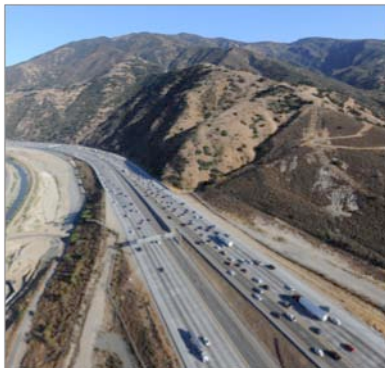
Toll Road Entrance, State Route 91
