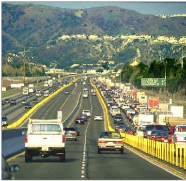
State Route 91 and 91 Express Lanes
