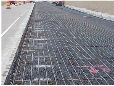
Continuous Reinforced Concrete Pavement
