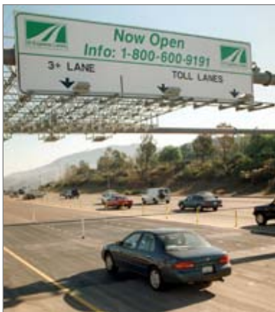
Transponder Plaza, 91 Express Lanes
