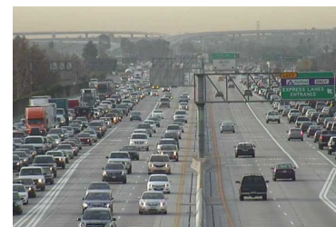
At-grade limited access configuration on LA Metro ExpressLanes
