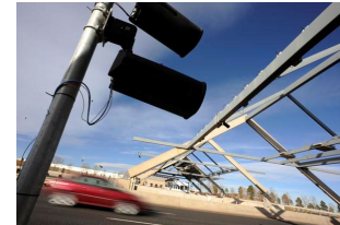
License-plate tolling equipment Craig F. Walker / The Denver Post
