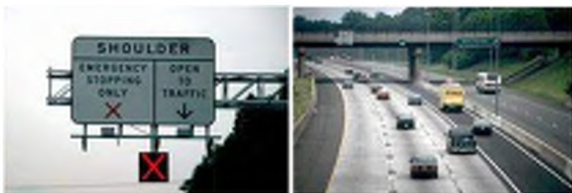
Figure 26: Lane Control Signal on I-66, Virginia Signage over right shoulder lane (left) with leftmost lane restricted to HOVs (right)
