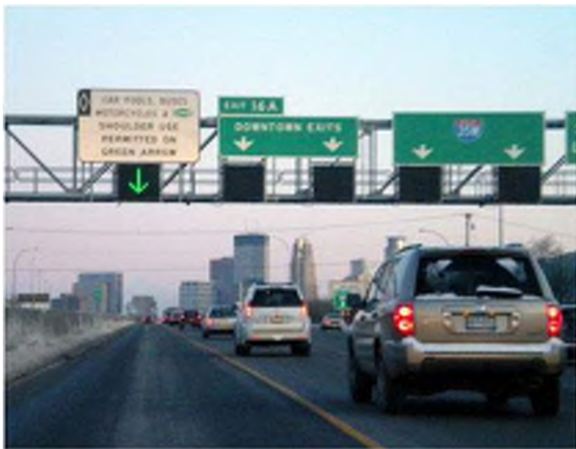
Figure 26: Lane Control Signal on I-66, Virginia Signage over right shoulder lane (left) with leftmost lane restricted to HOVs (right)
