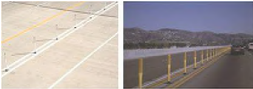
Figure 39: Examples of Pylons Placed in a Wide Buffer (left) and Narrow Buffer (right)
