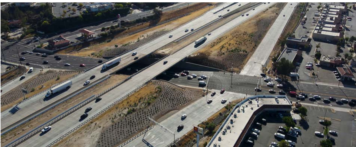
I-15 Railroad Canyon Road Interchange Project in Lake Elsinore. The new interchange opened in April 2022.
