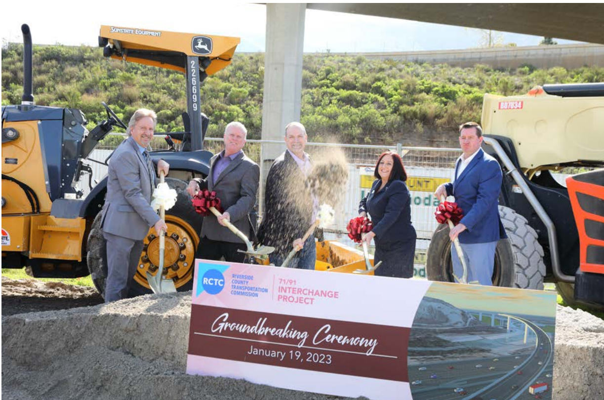
The 71/91 Interchange Project in Corona started construction in January 2023
