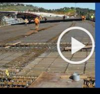
More than 6 million pounds of rebar were placed before pouring the concrete bridge deck
