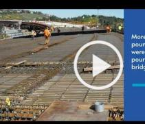
More than 6 million pounds of rebar were placed before pouring the concrete bridge deck
