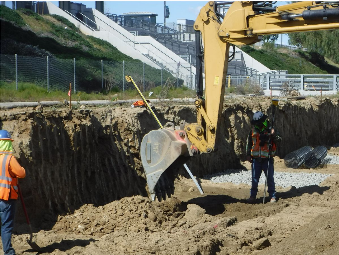
Due to heavy rains, crews remediated saturated soils and provided a solid, water-resistant base for new canopy foundations.
