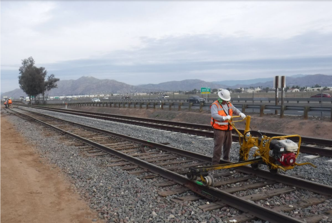
A construction worker uses a spike puller to remove old spikes from tracks.
