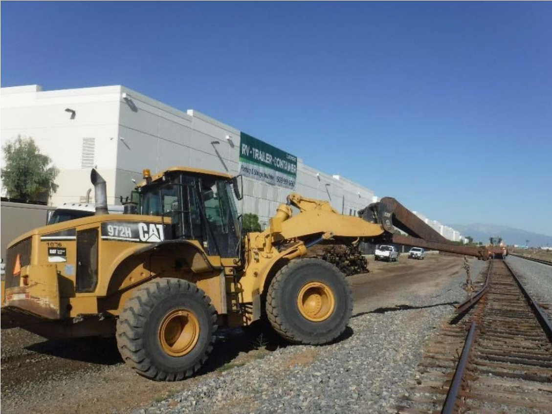
Existing tracks were removed in November 2022 to make room for upgraded tracks suitable for passenger trains.
