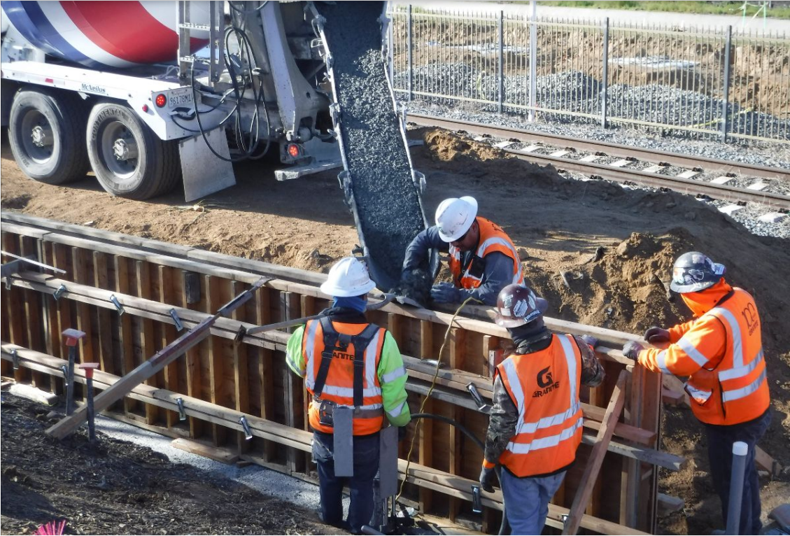
Crews pour concrete for existing platform extension retaining wall.
