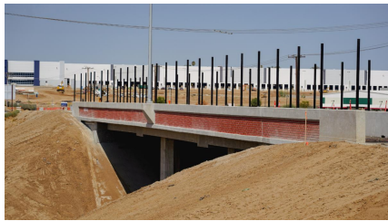
Fencing work on bridges.
