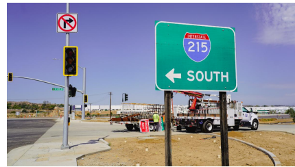
Crews installing new signs.
