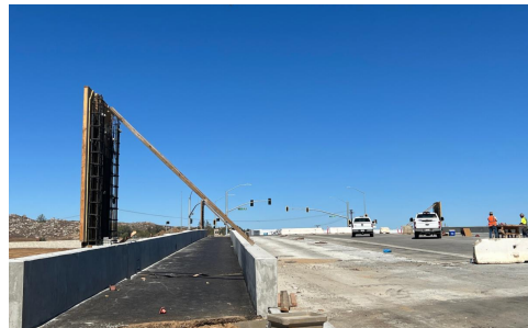
Progress on the equestrian path over the I-215 Placentia Ave. bridge.
