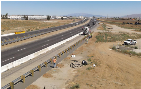
Crews pave around the new guardrail on I-215 below the Placentia Ave. bridge.
