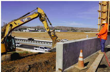
Final grading work around the new bridge.
