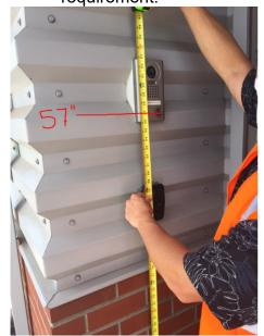
Replace with a compliant system with operable parts no higher than 48 inches per 308.3.1 and/ or 308.2.1.
