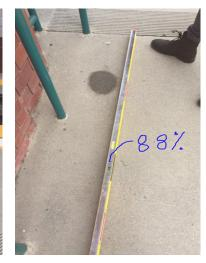
Remove handrails and replace the ramps with walkways no more than 1:20 slope.
