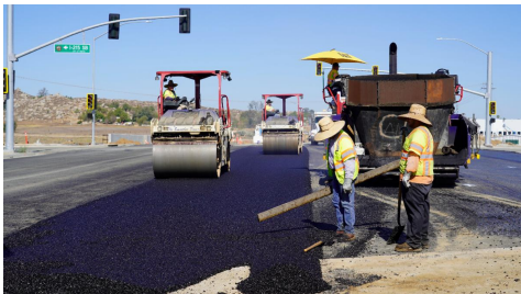
Crews pave Placentia Ave.
