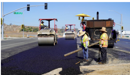
Crews pave Placentia Ave.
