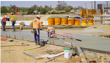
Crews have been pouring new sidewalks.
