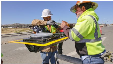
Electricians wire new signal lights.
