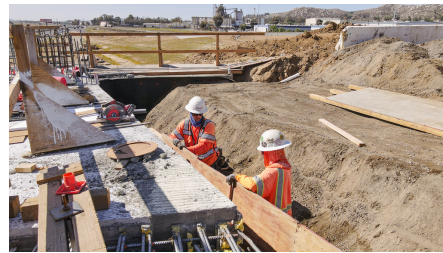
Crews work on the Placentia Ave. bridge over I-215.
