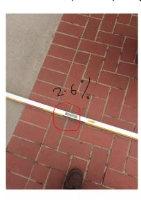
Repair cross slopes at paving features on accessible walking route or provide barriers at the inaccessible portions of the platform while ensuring alternate accessible routes
