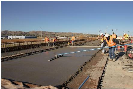
Concrete finishing work on the Placentia Ave. bridge over I-215.
