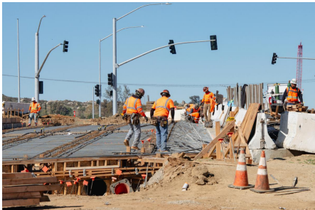
Crews work on the Placentia Ave. bridge over the railroad tracks.
