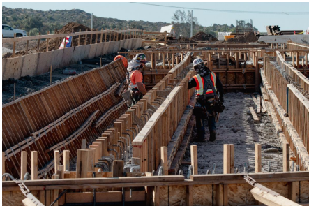
Crews work on the internal part of the Placentia Ave. bridge.
