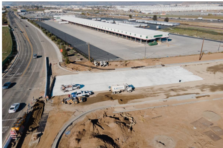
Concrete base has been poured on Placentia Ave. near Harvill Ave.
