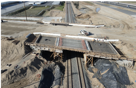
Placentia Ave. bridge over railroad tracks.
