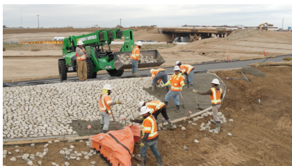
Decorative rock blankets are being installed.
