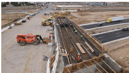
Crews place rebar for the widening of the Placentia Ave. bridge.
