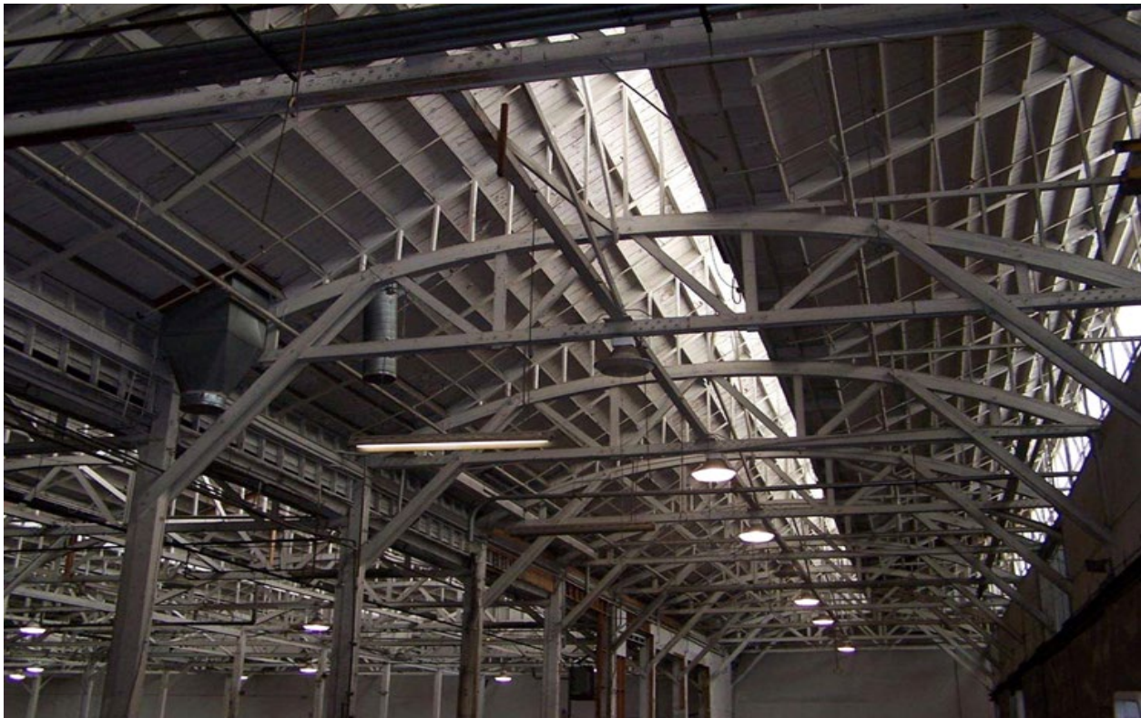
Figure 3-4. FMC Plant 1 Building A, Interior Bowstring Truss and Sawtooth Roof Looking West/Southwest
