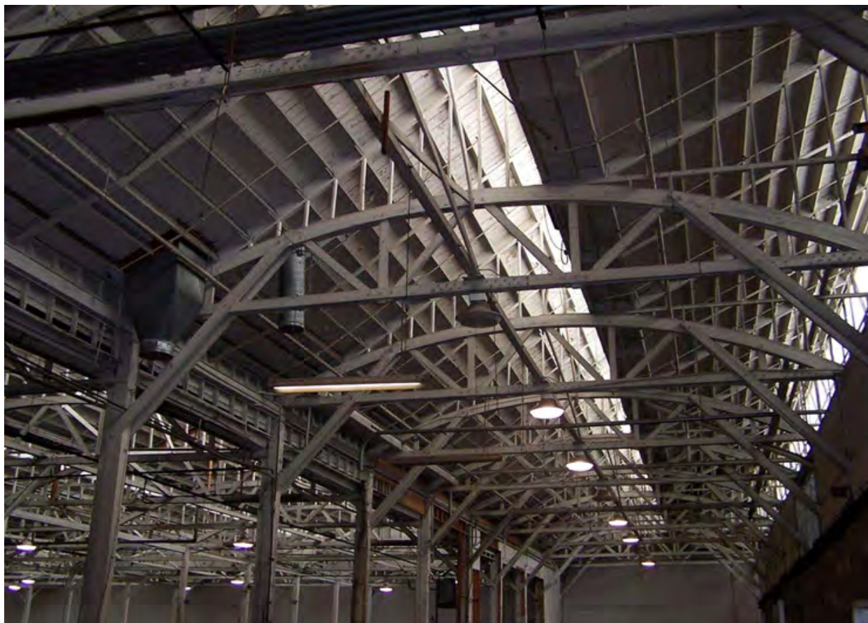
Figure 4-10. FMC Plant 1 Building A, Bowstring Truss and Sawtooth Roof Looking West/Southwest
