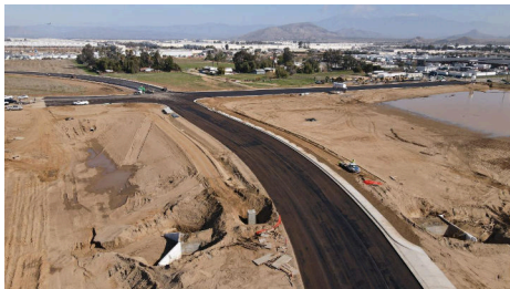
View of new E. Frontage Rd. alignment looking toward the Placentia Ave. intersection.
