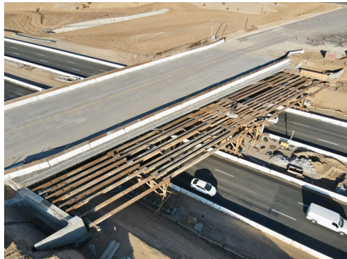
Steel beam support structure for bridge widening over I-215.
