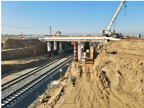
New columns constructed for bridge widening over railroad tracks.
