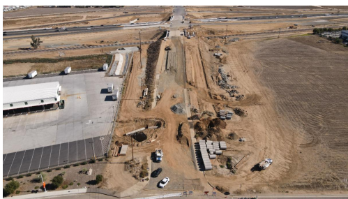
Storm drain work on Placentia Ave. near Harvill Ave.
