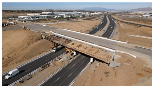
Progress of support structure for bridge widening over I-215.
