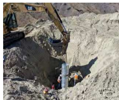
Crews continue to lay 15,000 feet of pipe for 123 drainage systems.
