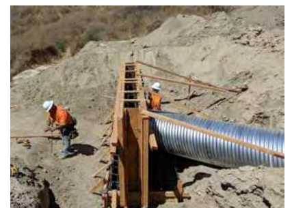
15,000 feet of pipe for 123 different drainage systems are being installed.
