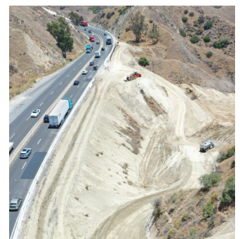
Excavators are beginning work to remove 2.1 million cubic yards of dirt from the hills next to Route 60.
