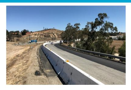
Crews recently set k-rail and completed shoulder pavement strengthening along the 15 northbound to 91 eastbound connector for the first phase of construction work.
