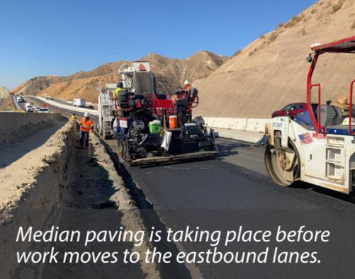
Median paving is taking place before work moves to the eastbound lanes.
