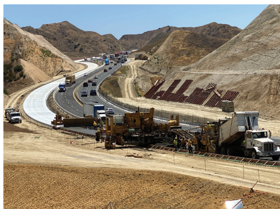
Crews are paving the westbound lanes. Read on to learn more about the paving layers.
