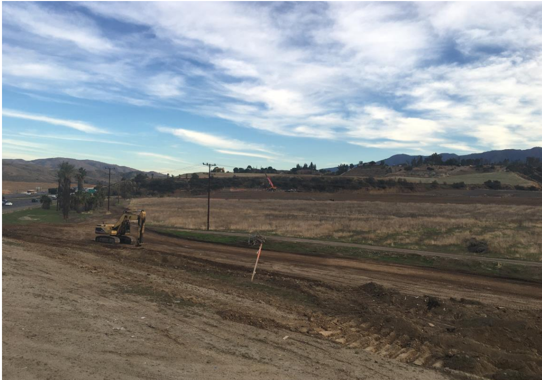
On Cajalco Road looking south. Southbound lanes of Interstate 15 are on the left side of photo.
