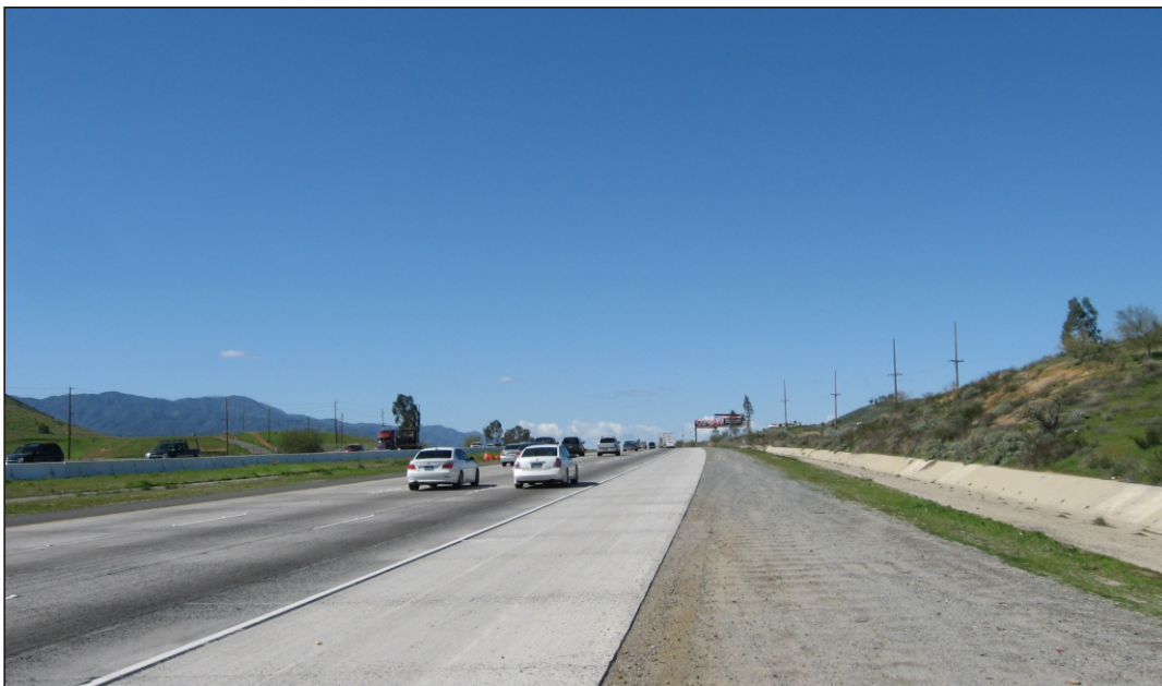
Key View 10: View facing north toward the future Franklin Street Interchange. The photograph is taken from the I-15 northbound lanes.
