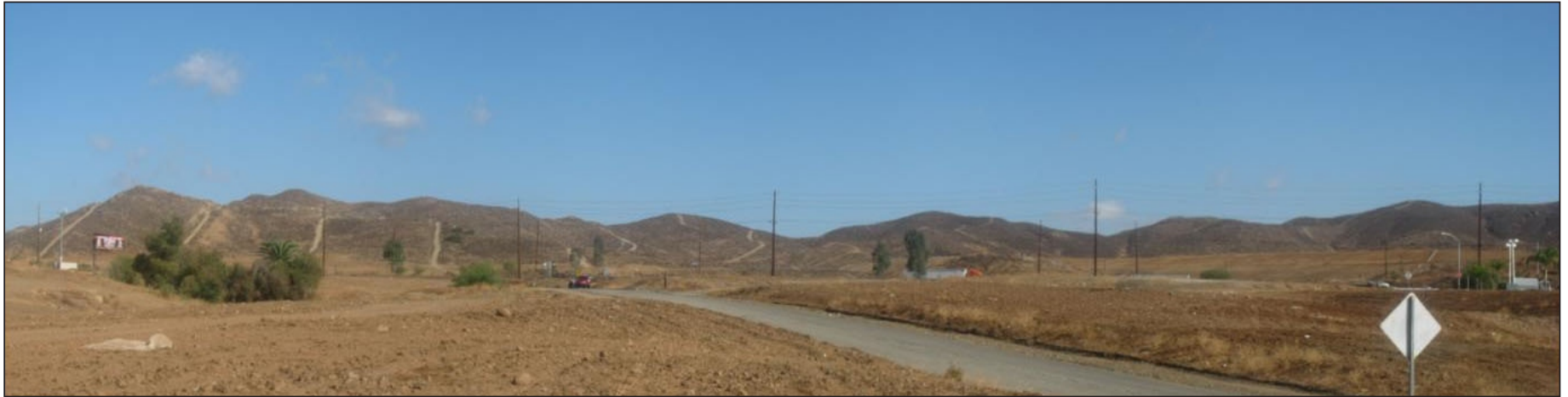
Existing View of Franklin Street Overcrossing, looking north.
